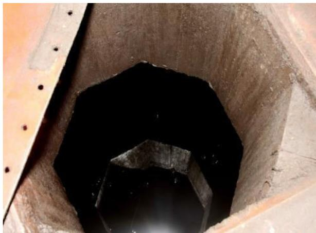
Fig 4 B: Man-whole of contaminated PCB oil with direct leachate into the Lagoon
